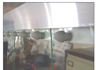
Photos above demonstrate the use of PVC strip curtains at Orange—BDP Data Center—Bristol and Yahoo in London.
